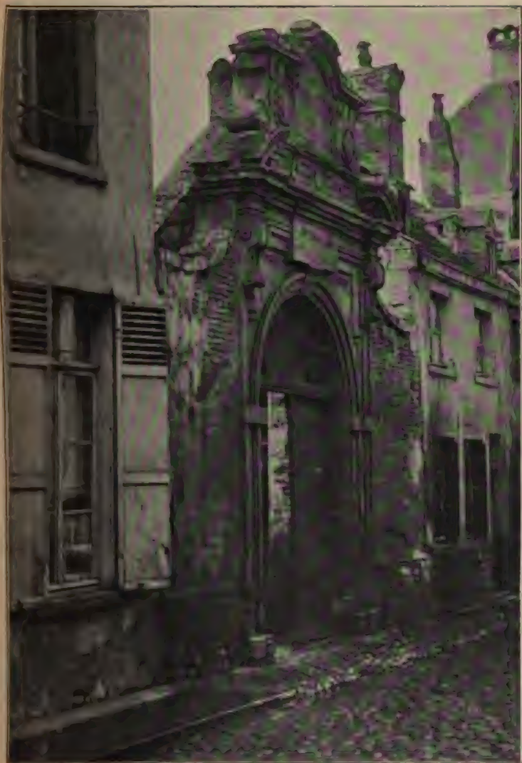
GATEWAY (NOW DESTROYED) TO THE GARDEN OF THE PENSIONNAT
